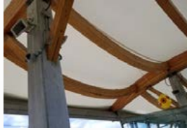
Edmonton Light Rail Transit Canada
